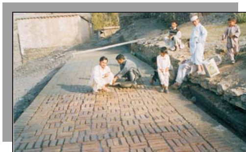
Community Productive Infrastructure Program
